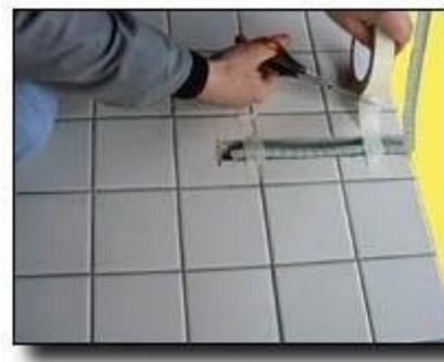
6. Unwind the cable reel totally, define the starting point and fasten the cable with the tape, after that unwind the reel to the end point (see picture).
